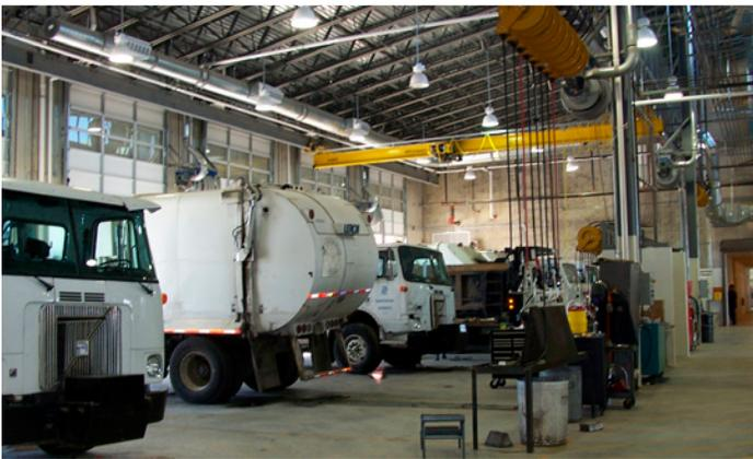
*Since the vehicle service center is not air conditioned, efficiency gains to meet LEED requirements are achieved by reducing winter heating loads rather than summer cooling loads.*
