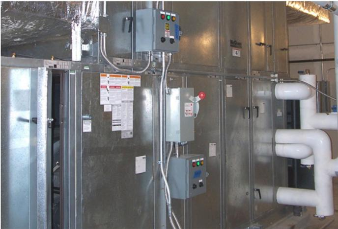
One of three large Daikin Vision air handling units installed for the vehicle service area
