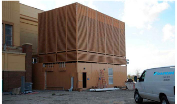
*A Daikin pre-fabricated modular central plant (MCP) complete with cooling tower and centrifugal chiller system*
