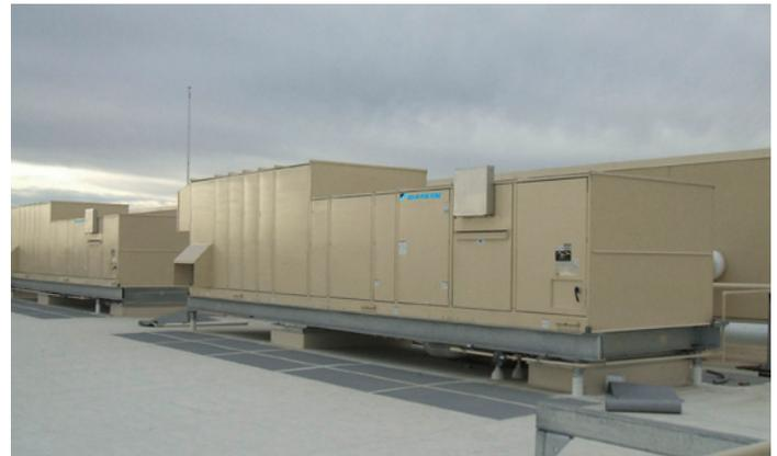
*Daikin RoofPak rooftop air handling units incorporating energy recovery wheels provide air to 344,000 sq. feet of space*
