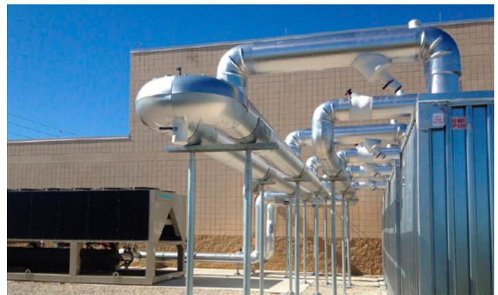
*The 265-ton Daikin Pathfinder air cooled chiller with premium efficiency is used as a "swing" chiller to shave demand by creating ice at night in conjunction with a FAFCO ice storage system.*
