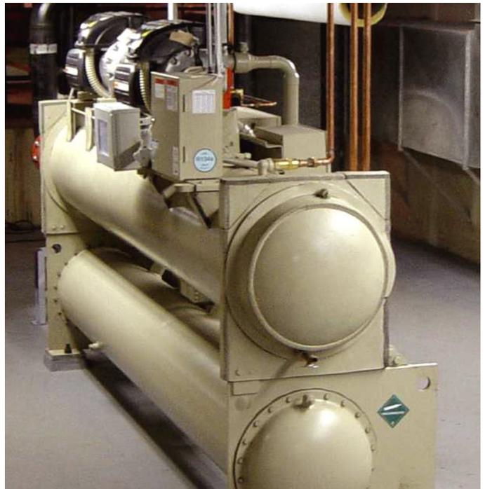
The two compressors of the Magnitude chiller operate on a common refrigerant circuit, improving system reliability.
