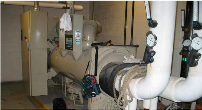
*Routine maintenance for one of two 275-ton Daikin water cooled centrifugal chillers.*
