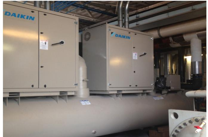
Six 1000-ton Magnitude chillers are among the new Daikin equipment serving the cooling needs for the airport's expanded terminals.
